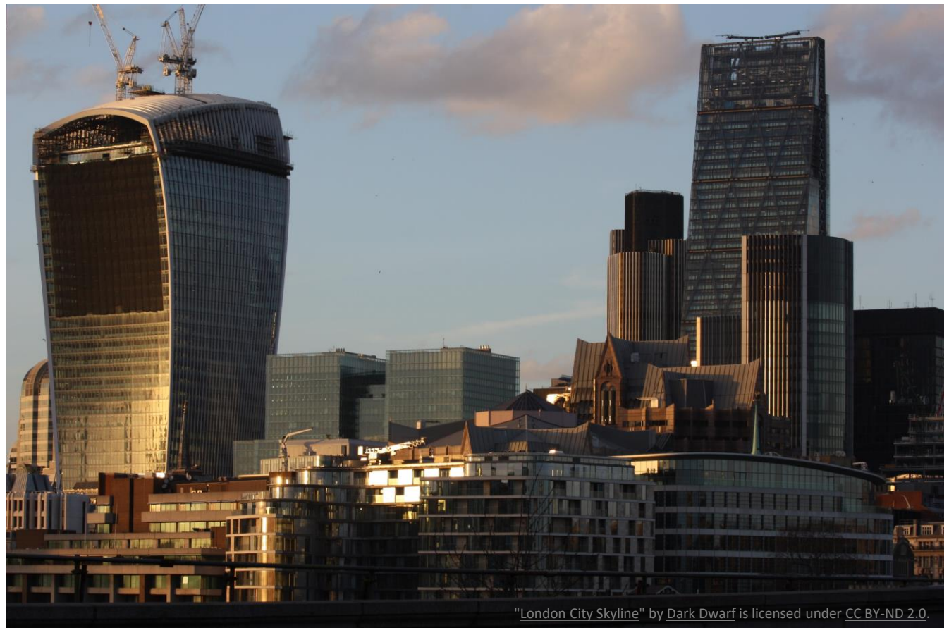
Figure 3.1: The City skyline viewed from across the Thames.
